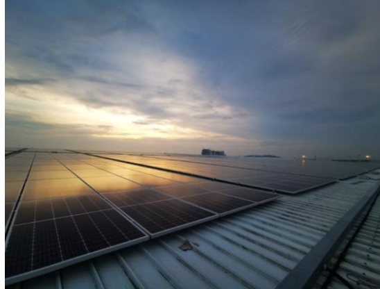
VAT Manufacturing Solar PV Installation - Side Profile
