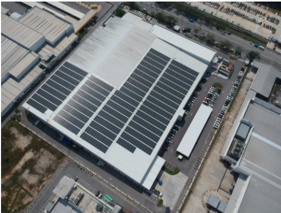
VAT Manufacturing Solar PV Installation - Aerial View
